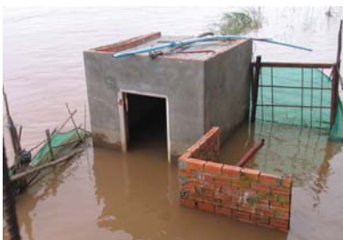
This is a photo of our back toilet - under water!
